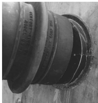
3. Place the Century-Line® Sleeve on the end cap. When field cutting non standard CS sleeve lengths, the sleeve and endcaps total length should be one-fourth (1/4") longer than the thickness of the wall. Cut with a hand or power saw.
