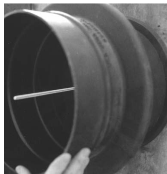
Place the sleeve over the end cap nailed to the form.
